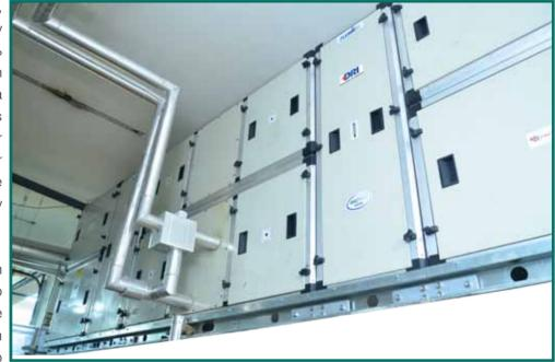
allows using DOAS (Dedicated Outdoor Air System) units for air handling with integrated energy recovery and moisture removal. As the primary air volume is reduced, the supply air needs to be dehumidified to become dry enough to carry out all internal moisture loads. This can be ensured with **DRI Ultima**, where double-wheel with cooling coil is able to remove enough moisture from primary air.
