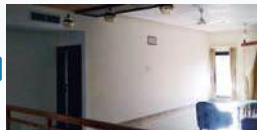
Residential Cooling Installations
