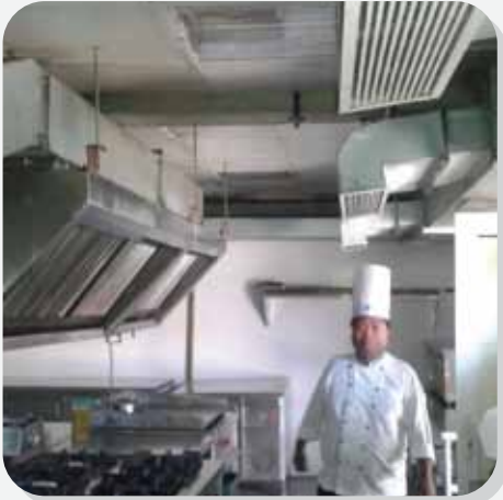
Kitchen & Restaurant Cooling
